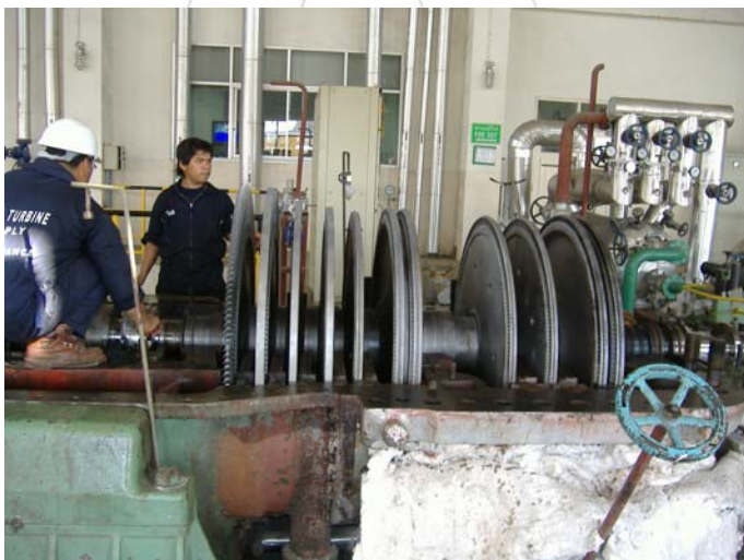
Major overhauling steam turbine generator 7500 kW. Of United paper.
