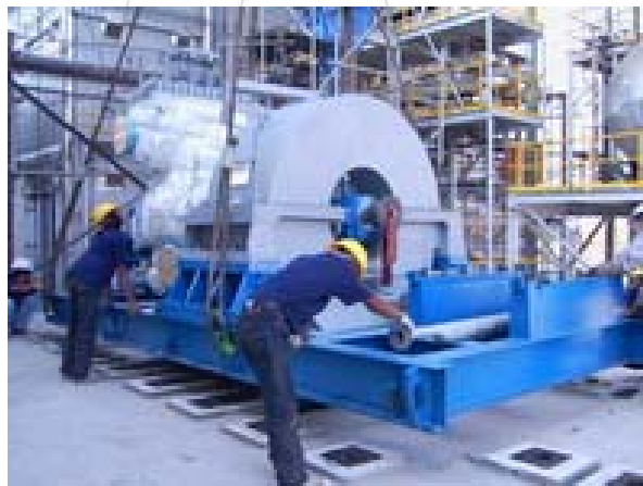
Steam turbine generator 9900 kW. Installation of Kaona power supply.
