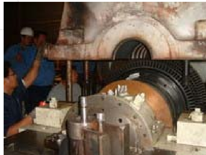
Overhauling steam turbine generator 12000 kW. Of Danchang BIO power.
