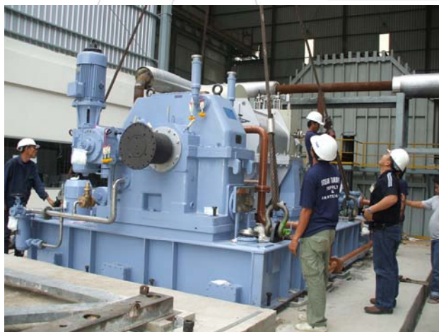
Steam turbine generator 8000 kW. Installation of Kaona power supply.
